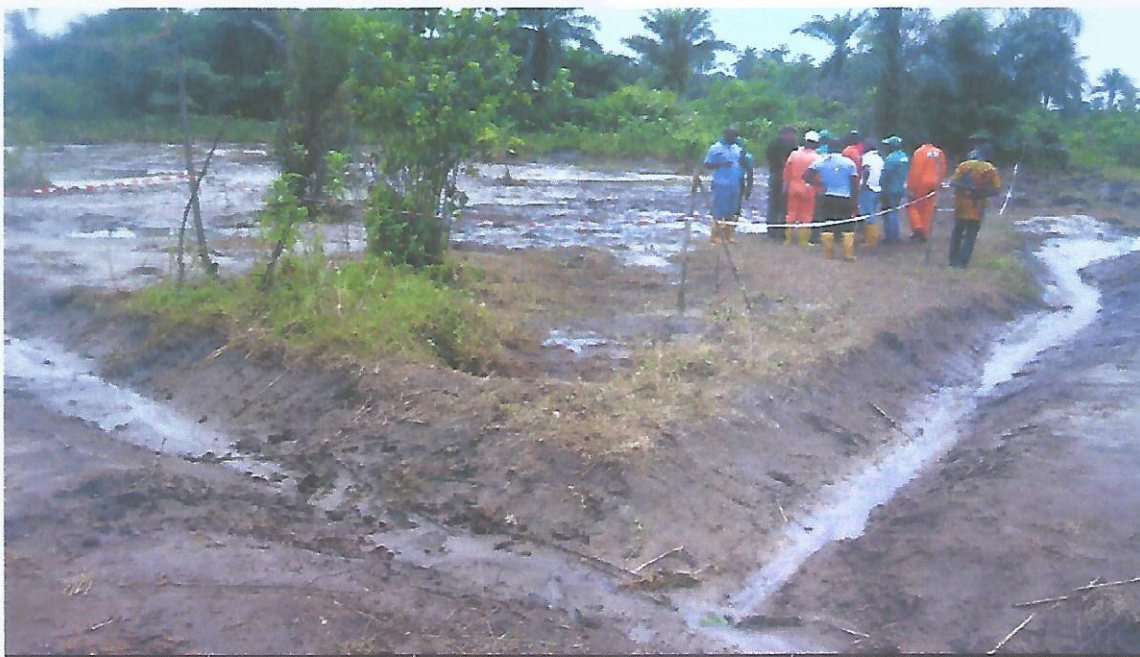
Figure 2. Cleared and demarcated site with trenches for diverting run-off
