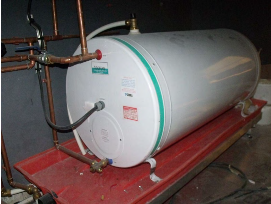
Figure 5-18: Hot Water Cylinder
