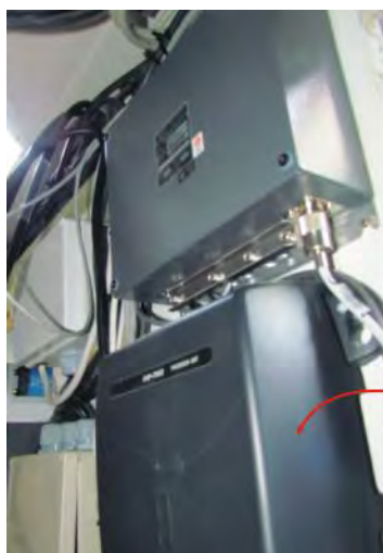
Figure 2-10: FAP-7002 Processor Unit Location
