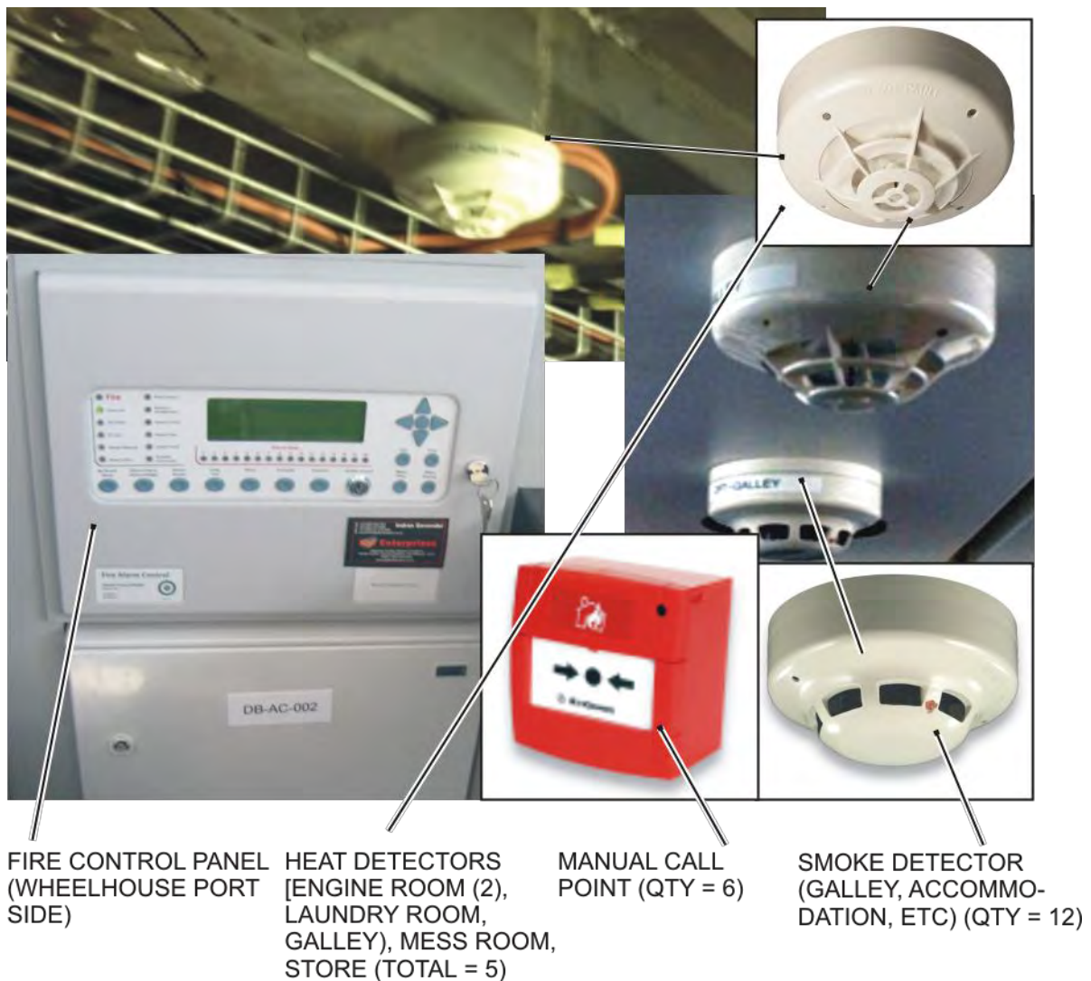
Figure 3-2: Fire Detection System Components
