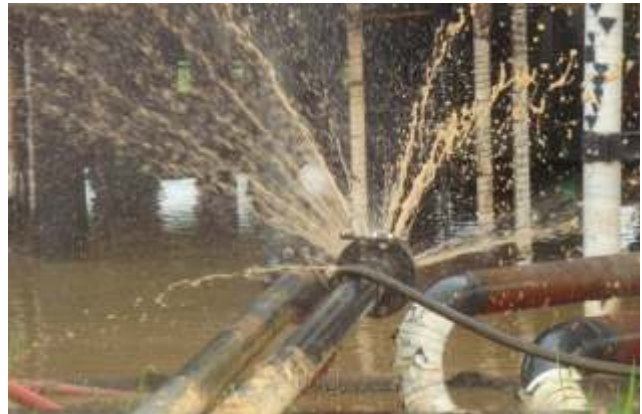
Flushing of complete 4" line 6 Nembe 3-Shell project
