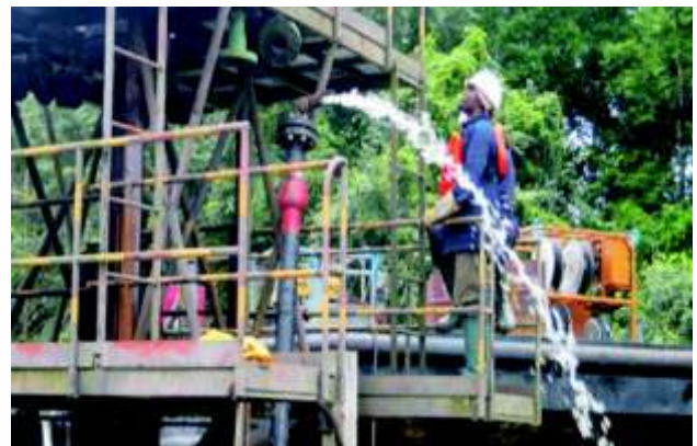
Flushing of completed line in readiness for pressure Testing of 6" line Azazuama to Tebidaba-32km Project executed for Nigeria Agip Oil Company.
