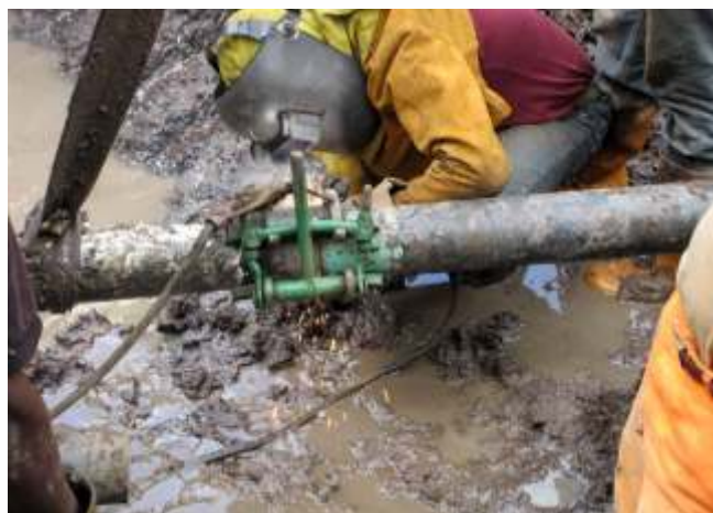
Fitting and tack welding of 6" line in readiness for Full butt of 6" inches Nembe South E and F-32km Project for Nigeria Agip Oil Company Limited.
