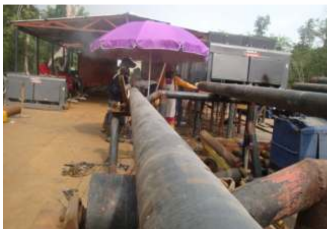
Radiography operations of welded 6" Ogboinbiri to Tebidaba 39km pipeline project for Nigeria Agip Oil Company Limited.
