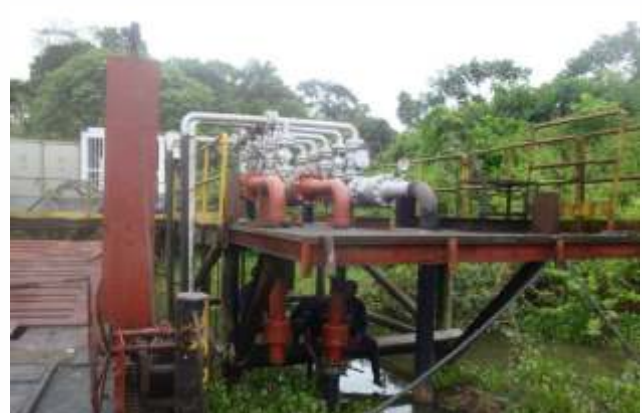
Installation of 6" riser for Tebidaba well for 14 Nigeria Agip Oil Company Limited.
