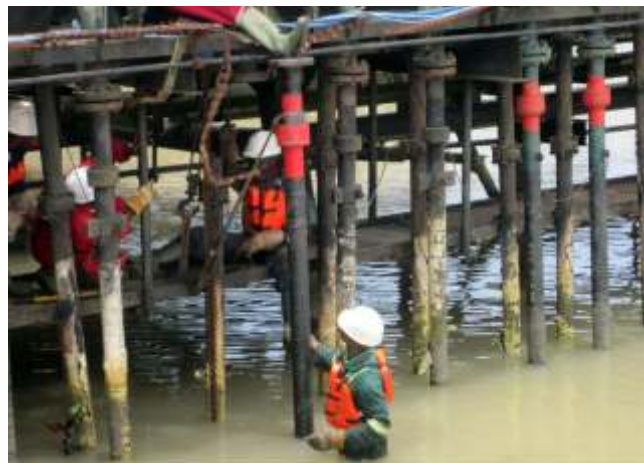
Installation of riser at production manifold for Nembe 3 flow station-Shell project.
