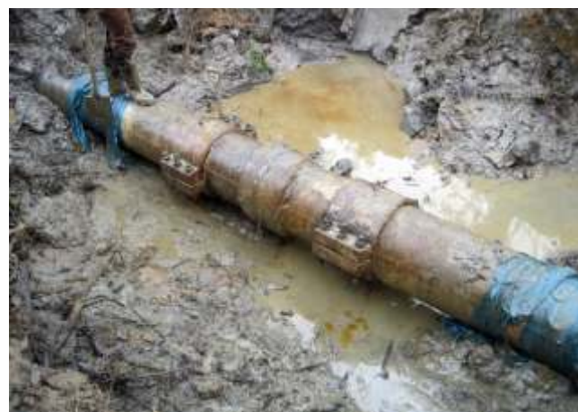
Leak repair by clamping of 18" Tebidaba brass line for Nigeria Agip Oil Company.
