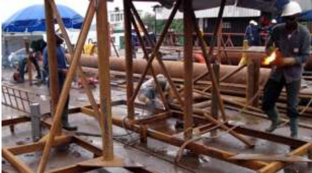
Welding operation for 6" Osiama line-15km Executed for Nigeria Agip Oil company.
