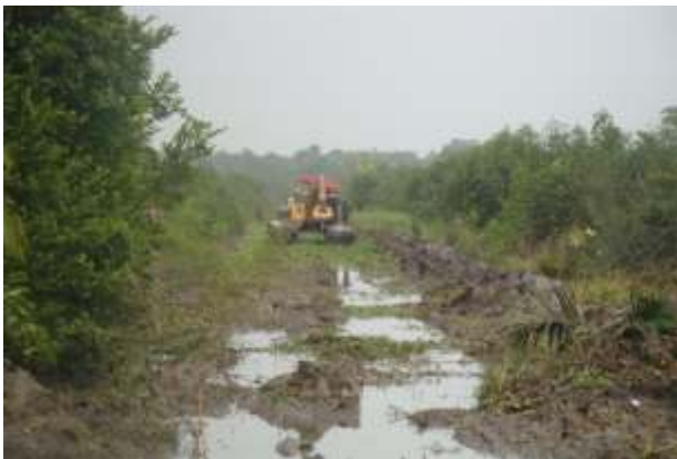
Excavation of ROW for installation of pipeline for Santa Barbara Shell project
